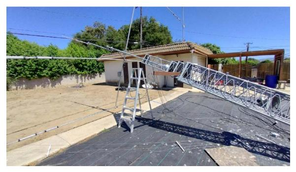
Now it was time to raise the tower and test my new antenna at height. Unfortunately I had forgotten to remove the red 2x4 before raising the tower to its vertical position and now there was too much weight resting on the 2x4 for me to remove it safely, so down came the tower again.
