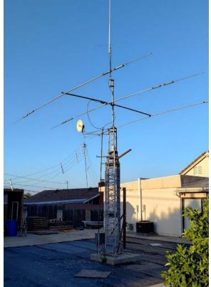
After removing the 2x4 the tower was returned to its upright condition and extended to its full height.
