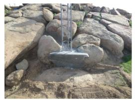
I had trouble with one tower bolt not going in. There is a small galvanized flake slightly blocking the hole. When I go up next I will bring a drill and clean out the hole and insert the last bolt.
